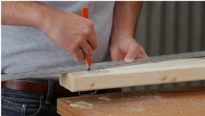
Mark the lines on the 2x4s. Measure and mark the 2x4s as shown in the diagram.
