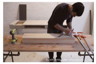
Lay out the holes. Use a pencil to mark the hole locations on a board. Make sure you leave about 2" between the flower pot holes and about 1" between the rope holes and edges of the board.
