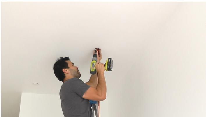
Install the Rack I wanted to make sure that I was attaching the rack to one of the beams behind the drywall of my ceiling, so I used a stud finder to locate it. I used my Phone Works stud finder to find the center of the beams. Then I screwed 3/4" copper loops on either side of the T-fitting.
