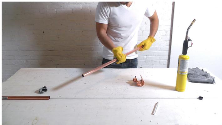
Clean + Prepare the Copper I cleaned the copper with steel wool and used a wire brush to rough up the ends that are going to be soldered.
