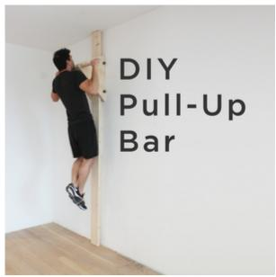
This DIY Pull up bar doesn't need a doorway and can serve as a work out station for additional exercises. It is made from 2x4s, 2x6s, ¾" plywood and some iron pipe fittings. I was very carful to make sure that the structure was securely fastened to the wall to avoid injury. I consult a personal trainer, fitness expert, and doctor attempting any sort of fitness activity.
